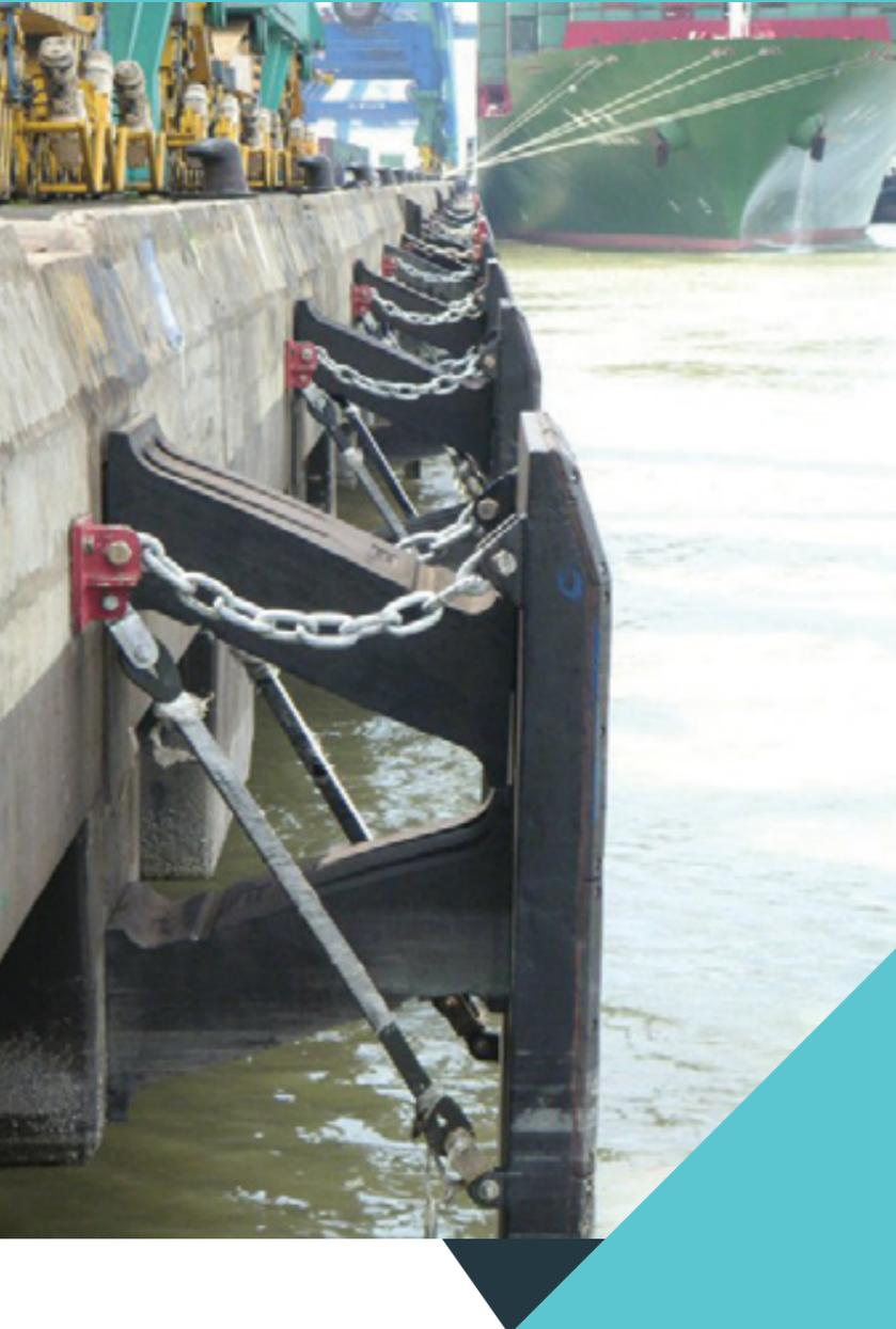
Leg Fender which is also called Unit Element Fender or Element Fender is a high performance, modular system. It has been widely used across the world for decades. The construction of the Leg Fender is simple but very strong and durable. They can provide good protection for piers and docks.
