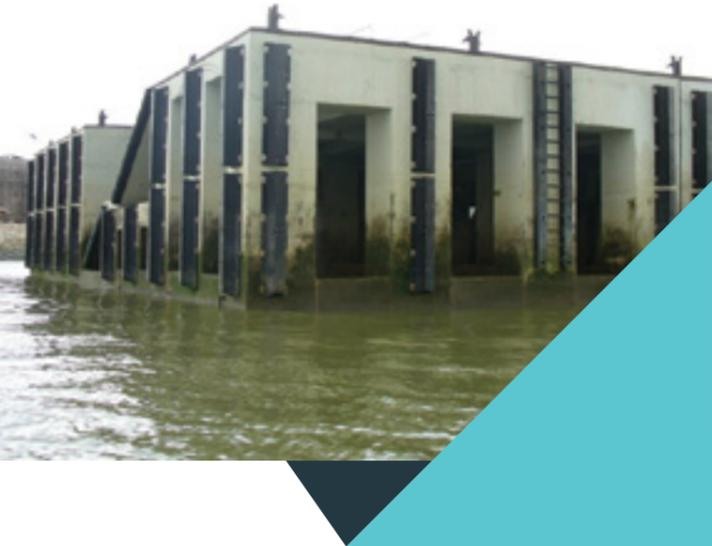
Rubber Ladders are very robust. They are flexible to reduce accidental damage and protect the wharf from small craft berthing. The modular Rubber Ladders are durable, tough and also have high corrosion resistance. They can withstand most accidental impacts from smaller vessels. They can function as fenders for small boats and also as ladders.
