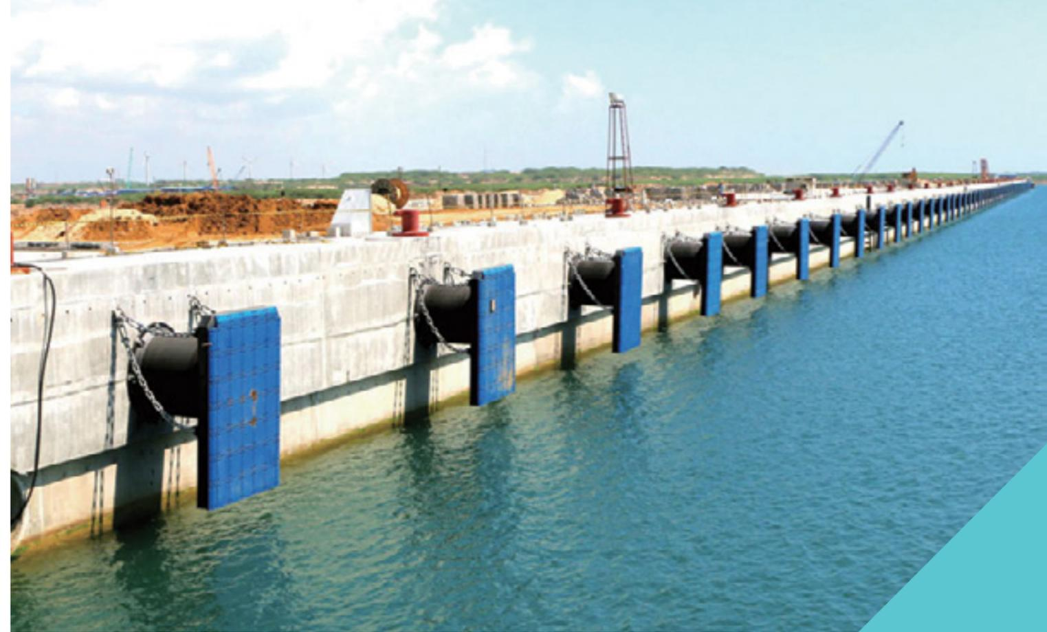
The Super Cell Fender is improved over the ordinary type. It is the most commonly used fender in the world. The circular mounting base of the Super Cell Fender makes it an extremely stable fender type.
