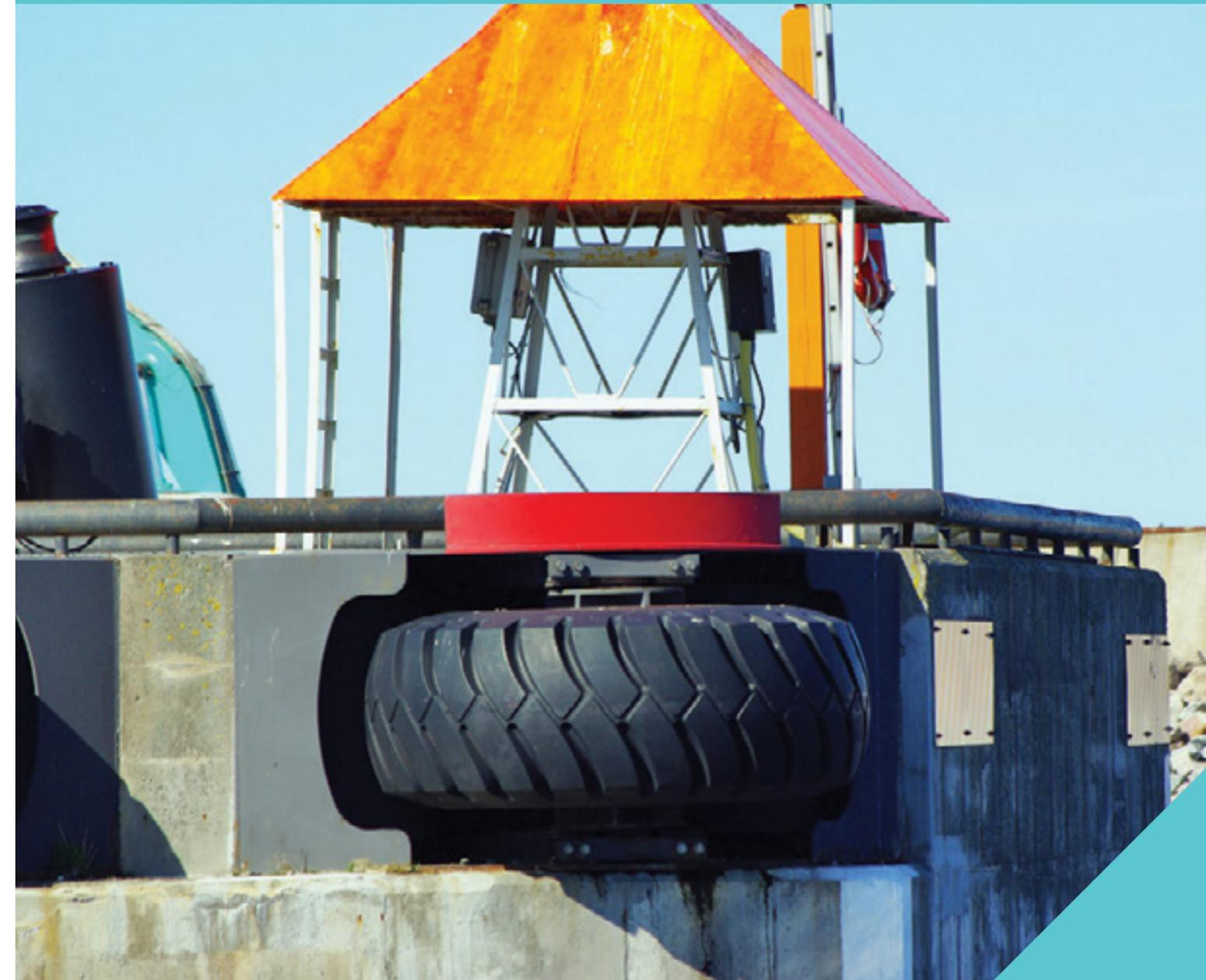
Roller Fenders are widely used on exposed corners to help ships manoeuvre into berths and narrow channels such as locks and dry-dock entrances. There are two types of Roller Fenders and each has its own features and applicable conditions.
