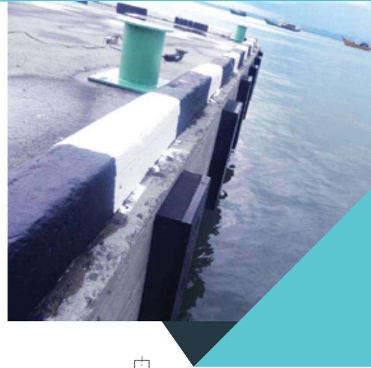
HD-PE Sliding Fenders are the perfect substitutes to quay wall protection due to the advantage of low friction and better wear resistance. HD-PE has the characteristic of non-splitting or non-decay and is totally resistant to borers. HD-PE is easy to machine and install onto concrete, steel or timber substrates. HD-PE is fully recyclable after its working life, and is a cost-effective alternative to tropical hardwoods,
